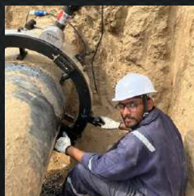
Pipe Cold Cutting
